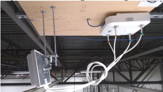
Figure 4: All-thread method
